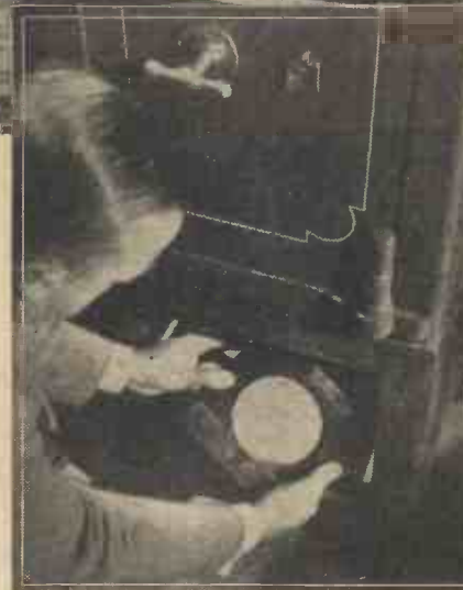
These illustrations show how a shopkeeper protects his safe by placing a Philophone underneath it where it cannot be seen. Should anyone approach the safe, the slightest noise will be intensified in the master unit, in his bedroom upstairs, sufficiently to awaken him.
