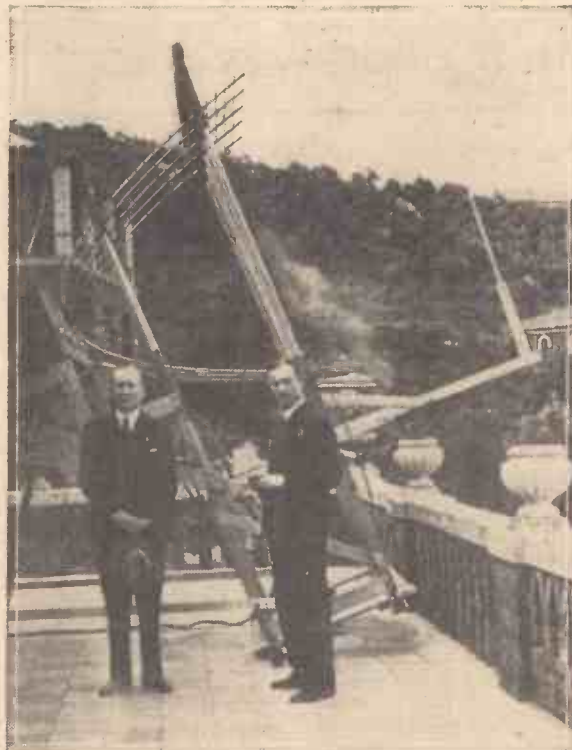
Fig. 2.—This illustration shows a commercial beam or reflector transmitting aerial and clearly indicates the method of assembly.
