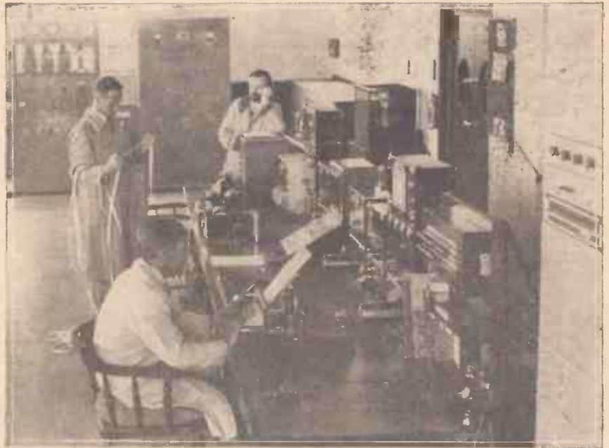
The control table for the transmitters at the new Police Radio Station at West Wickham, Kent.
