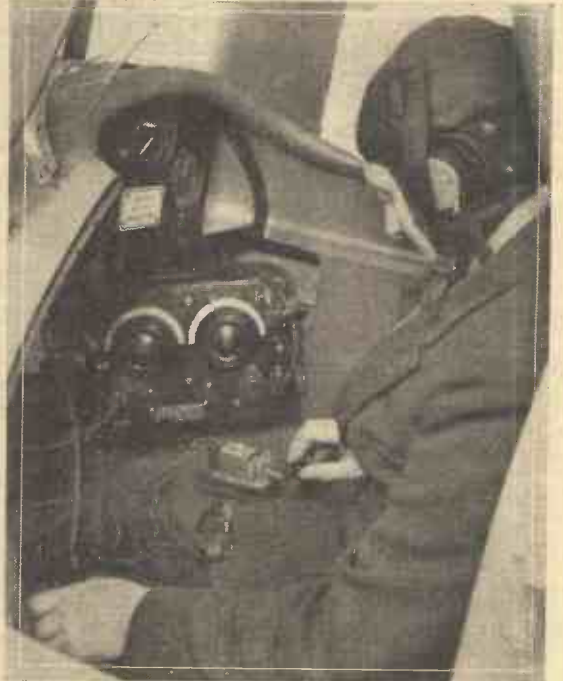
Marconi transmitting and receiving equipment installed in the observer's cockpit of the Scotland Yard Autogiro. The receiver is immediately below the dashboard, and the transmitter, which is worked by the morse key strapped to the observer's leg, can be seen above his left hand.
