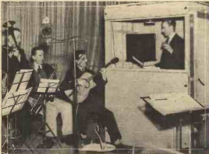
Ray Noble, the dance music composer-conductor, used for the first time recently a new invention when making records in the "His Master's Voice" studios. He conducted his orchestra from a sound-proof box, and heard their playing through a loudspeaker at his side. Thus he was able to ensure that all the instruments were perfectly balanced and managed to obtain effects that have not been possible hitherto.
