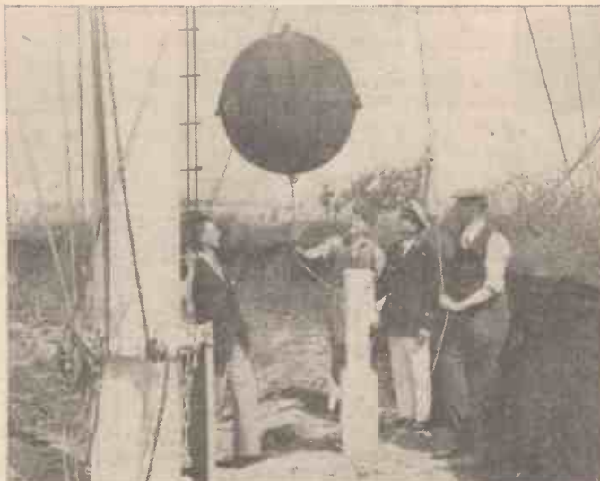
The Naval Time-Ball Signals, which have been in constant use since 1888 at Mount Wise, Devonport, Devon, giving the official time to the naval ships and mariners, have, by Admiralty orders, to be dismantled, the more up-to-date method of time signalling by wireless now being in use.
