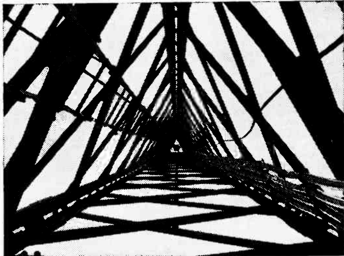
This is an interior view, looking upwards, of the 250ft mast at Llandrindod Wells, central Wales, for which EMI Electronics Ltd. have supplied a turnstile aerial array to the British Broadcasting Corporation. This is one of five new stations which the BBC is building to extend its television and sound services and to improve reception in the fringe areas.
