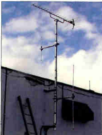
A DAB single dipole aerial fixed to the TV aerial mast. The DAB aerial is the short vertical dipole on the left. In many cases this is the correct DAB aerial for a communal aerial system, a directional aerial being unnecessary. In fact the proximity of the mast will unavoidably give the aerial slight directivity.
