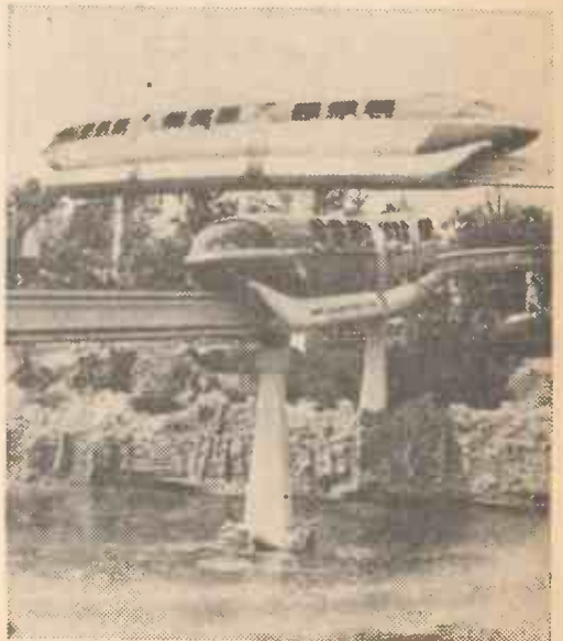
Part of the mile long Monorail track at Disneyland, California.
