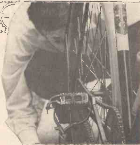
Fig. 2.—Sighting along the chain.
