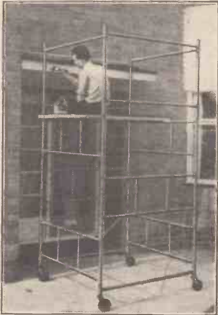
Scaffold kit in use.
