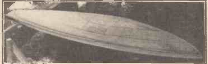
Fig. 7. (Right) — The male form is ready for the work of getting a very high polish. The smooth perfection of this finish will be repeated in the inside of the female form, and ultimately on the outside of the finished hull.
