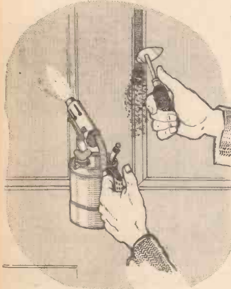
Fig. 1.—Use of blowlamp and shave hook.
