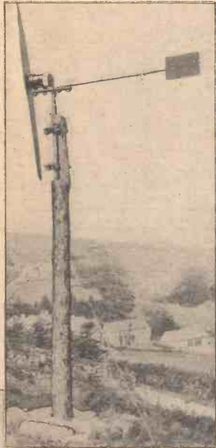
Fig. 3.—Showing methods of attaching dynamo to turntable described, and to a flat bar, as in the model illustrated.
