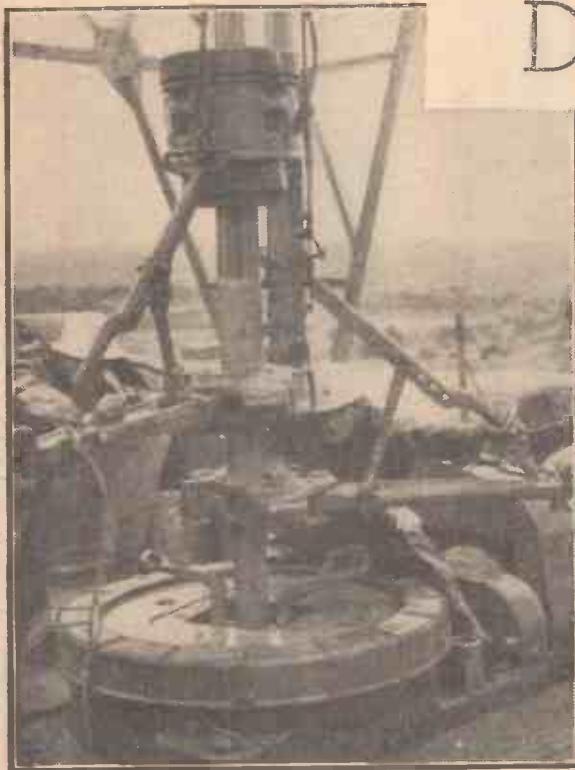
Drilling for oil at Arreton, Isle of Wight, where operations have already reached a depth of over 1,700ft. Illustration shows the connecting link on the drill being tightened.
