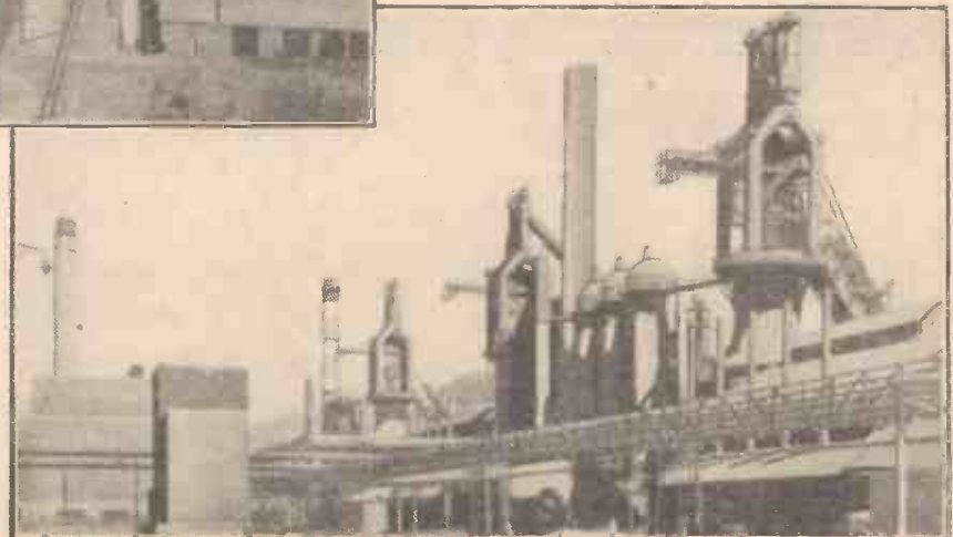
The Geneva plant's 1,100-ton blast furnaces; the 50,000-kilowatt power plant and switch house.
