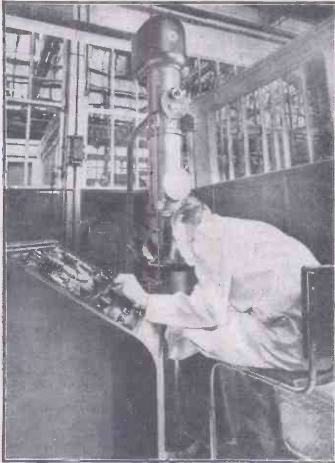
Fig. 6.—Metrovick new electron microscope in use.
