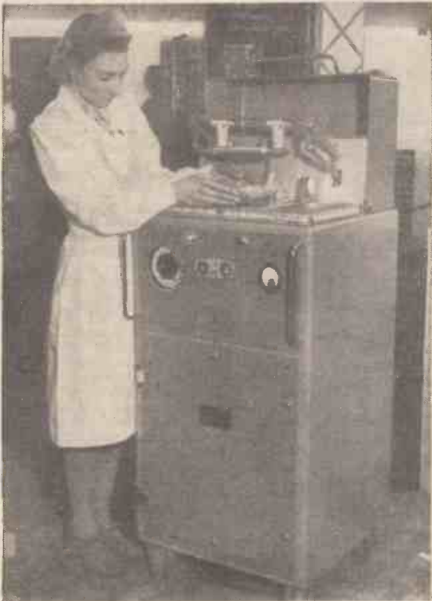
"Cooking by radio." In this cooker house current is transformed into radio-frequency current and focused directly upon the food. No heat is wasted, and the cooker remains cold.
