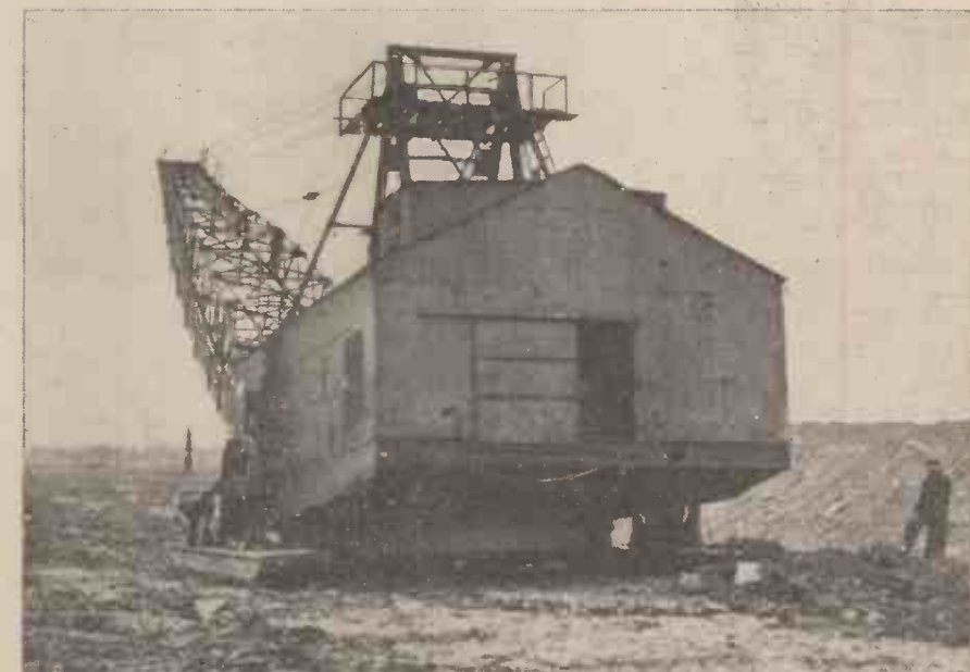
A rear view showing the Bucyrus Monighan machine about to "walk."
