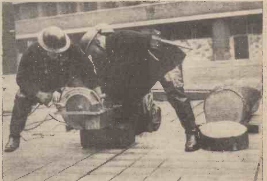
A demonstration of German fire appliances took place recently at London Regional H.Q. Our illustration shows British firemen operating a portable electric circular saw carried on a German Emergency tender. We have no equivalent in our fire service.
