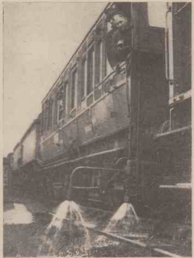
The L.M.S. Railway is now using a special "weed-killer" train for spraying a trail of poison along the entire L.M.S. system from Wick to Shoeburyness, and across Britain to Holyhead. The "weed-killer" train sprays on an average 70 miles of track a day. If left unattended, many of the tracks would become covered with weeds, but these are eliminated by the poison spray. The illustration shows the spray train in action in the Midlands.
