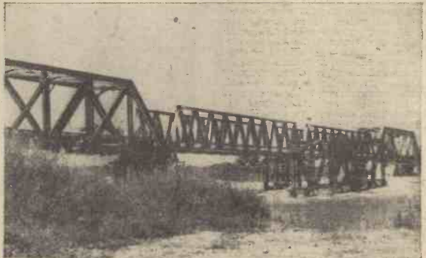
Sinthe Bridge ready for use. The two new centre spans, each weighing 70 tons, can be seen. They are supported by light steel trestles on reinforced concrete slabs.
