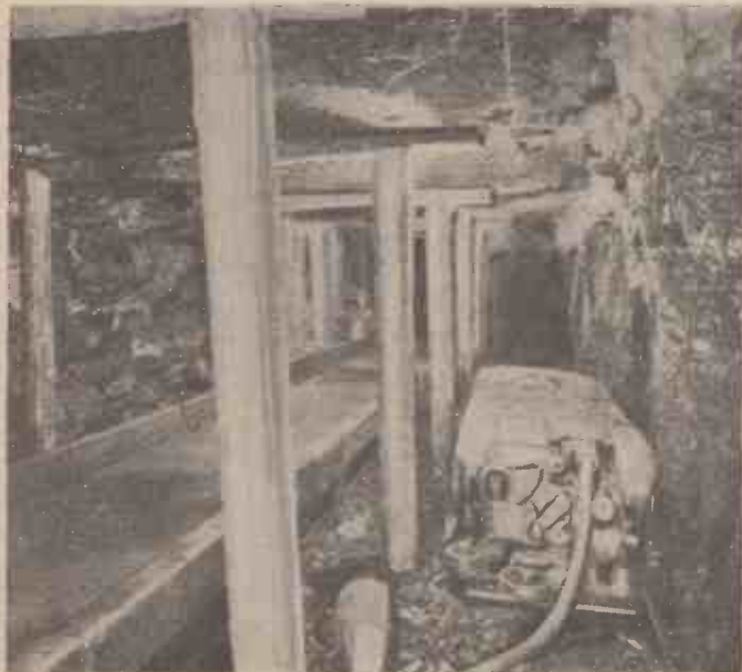
Cutting the face with an A.C. longwall Samson. The machine is hauled along by winding in the drum on the face side, the end of the rope being fixed by a prop. The face conveyor is shown in position ready for commencement of the loading shift.
