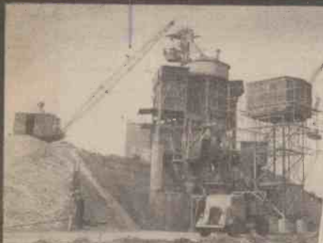
The huge mixing machine making concrete for the runways.
