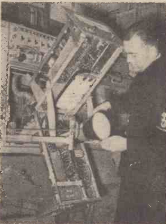
Radar in the Navy. This equipment was designed to provide radar-controlled fire at enemy planes, using the main A.A. batteries, in large modern ships. It can also control the main armament of a destroyer against surface targets. The modulator and receiver are similar to those used in the surface gunnery equipment.
