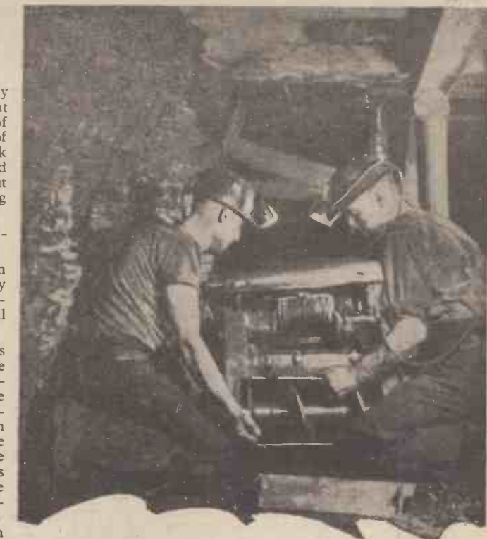
Side discharge gummer being fitted to machine at beginning of shift. The driving gearbox is seen bolted to the gearhead frame.
