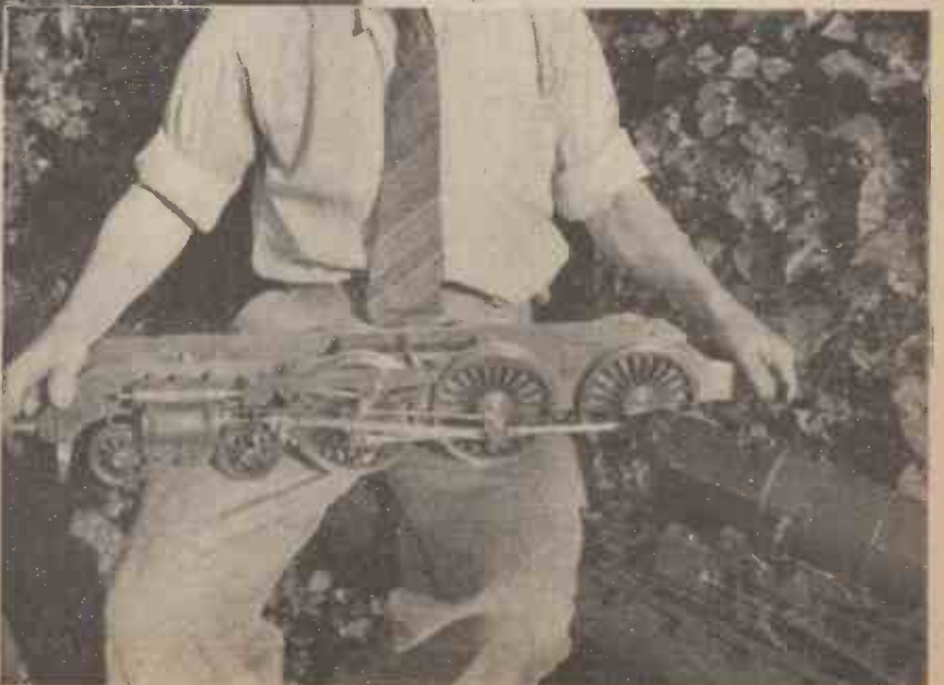
Fig. 3.—Close-up of the ¾ in. gauge "Royal Scot" chassis
