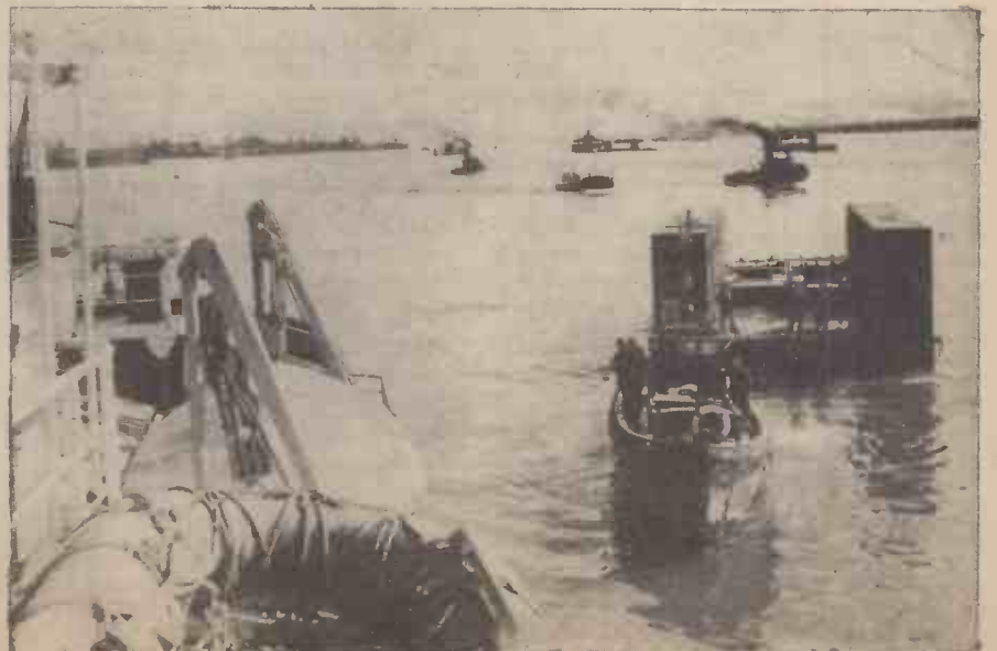
Attempts are now being made to seal off the breaches in the dykes on Walcheren Island. Parts of Mulberry Harbour used for the invasion of Normandy are being taken to Walcheren, and our illustration shows pontoon units being brought alongside tugs in Southampton Docks.
