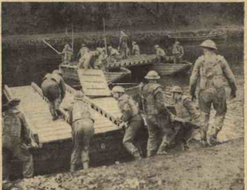
When Western Command War Correspondents visited a Royal Engineers training battalion recently, a demonstration was given of wet and dry bridge making. Our illustration shows a floating bay bridge being assembled during the demonstration.
