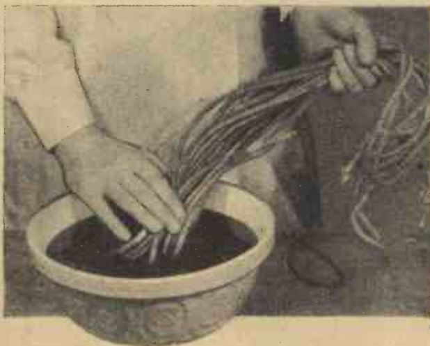
Chemically impregnating rope previous to its use in a damp situation. Woodwork and sandbags may be treated similarly, as described in this article. (Left.)
