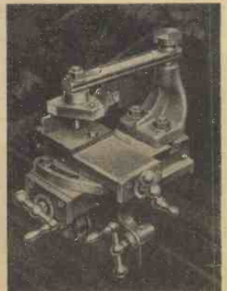
The Myford parting-off attachment.
