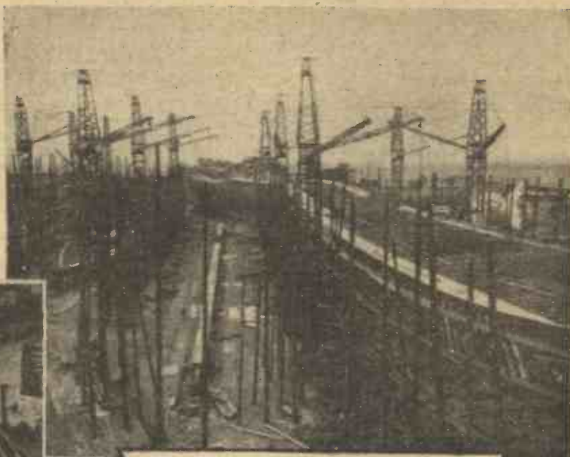
In the centre foreground is seen the keel of a new ship and on either side are vessels in different stages of construction with two new ships in the fitting-out basin beyond.
