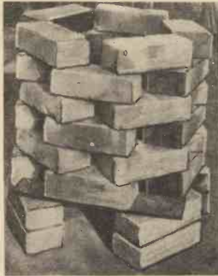
Fig. 1.—A small incinerator built with old bricks costing five shillings.
