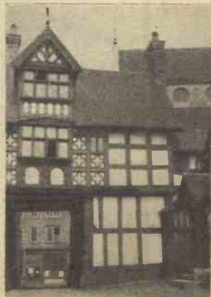
The Council House Gateway, Shrewsbury.
