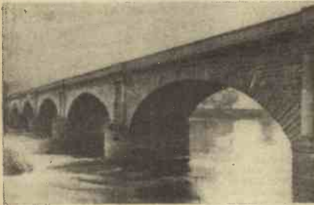
Rennie's first bridge, which he designed in 1799. It was erected over the Tweed at Kelso, and completed in 1803.
