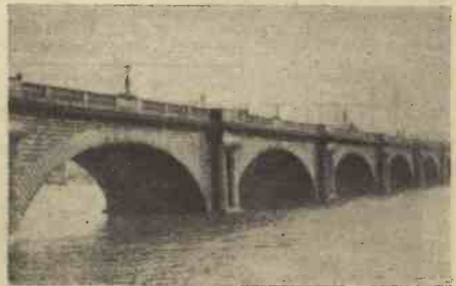
The old Waterloo Bridge, which was demolished a few years ago: It was considered to be Rennie's masterpiece, and was first opened in 1817.
