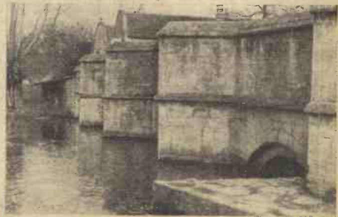
The old bridge over the Windrush, Burford
