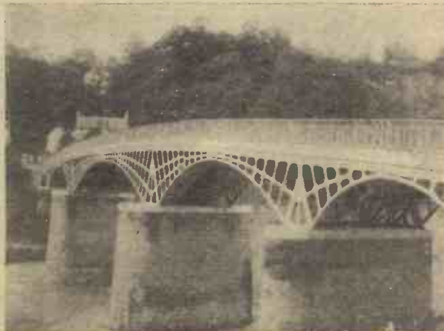
Rennie's cast-iron bridge over the Wye at Chepstow. Erected in 1817.
