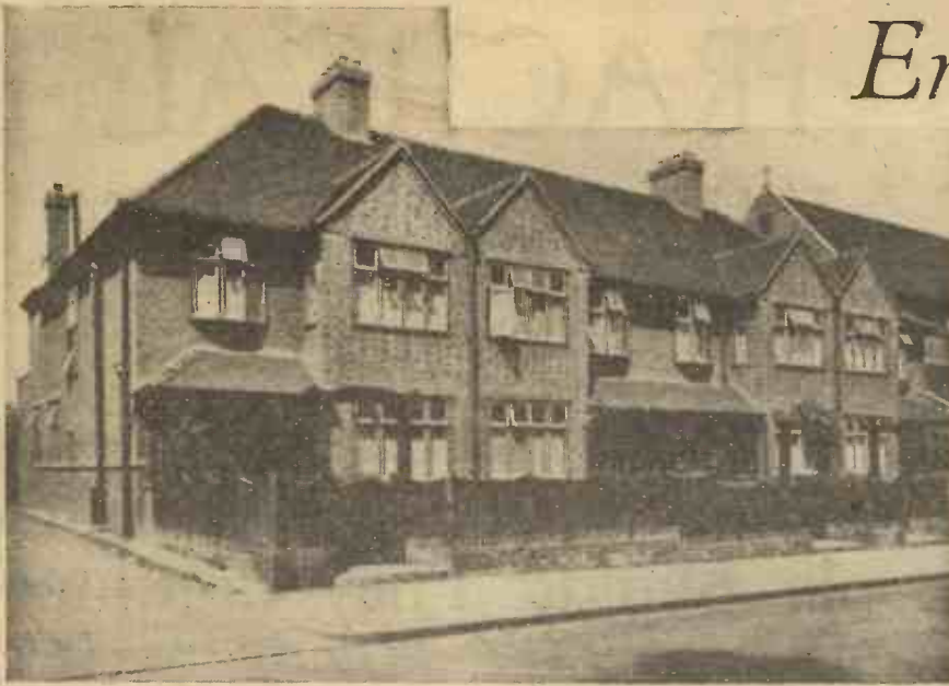
Fig. 1.—Typical pre-war houses similar to those which each weigh about 125 tons. Brick built, tiled roof, tiled bathroom and chromium-plated fittings.
