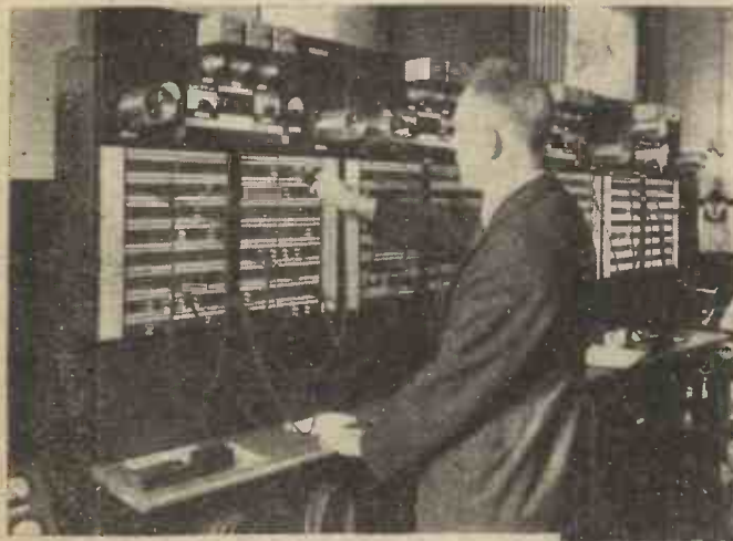
Testing lines at the C.T.O. (By the courtesy of the Postmaster-General.)
