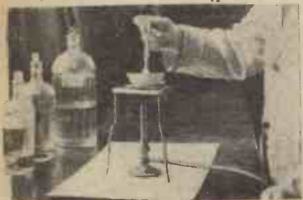
Making bakelite resin in the home laboratory by the interaction of formalin and carbolic acid.
