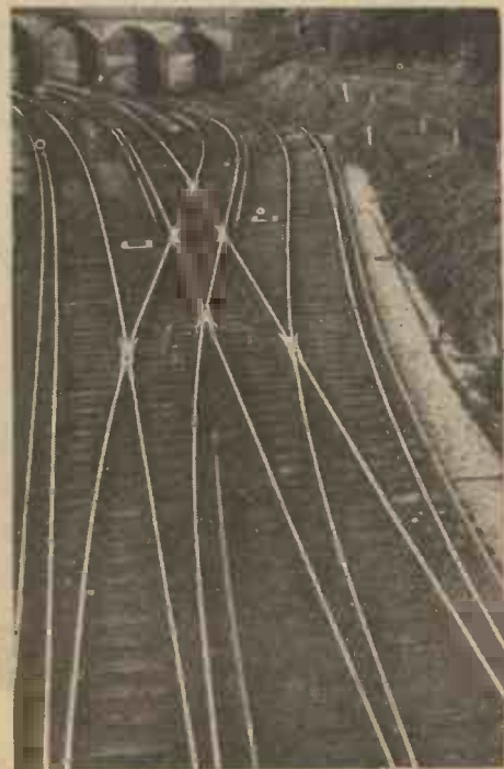
A busy railway junction in which the crossings are of manganese steel
