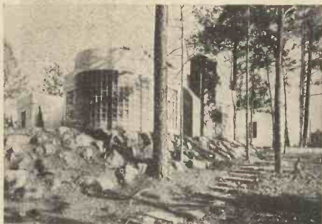
Fig. 1 (above). A dwelling house constructed with the new welded steel panels.
