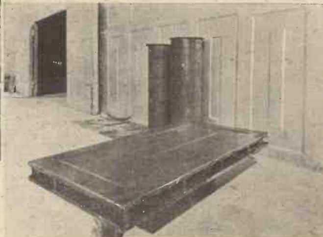
Fig. 2 (below). One of the "building blocks," or panels, showing the interior spacers.
