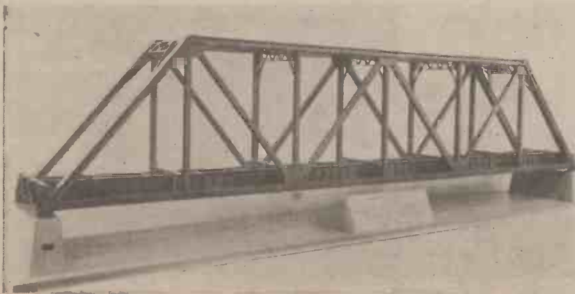
A realistic model of a 45-metre span bridge—scale 1 in. to 1 foot—as used on the Tientsin Pukow railway in China.
