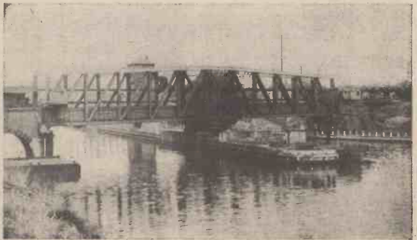
The modern swing-bridge which carries Brindley's original canal across what is now the Manchester Ship Canal.
