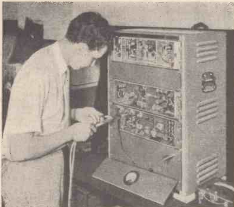
Fig. 1.— The two amplifiers with their equalisers and power supply are mounted in small portable cabinets as shown.
