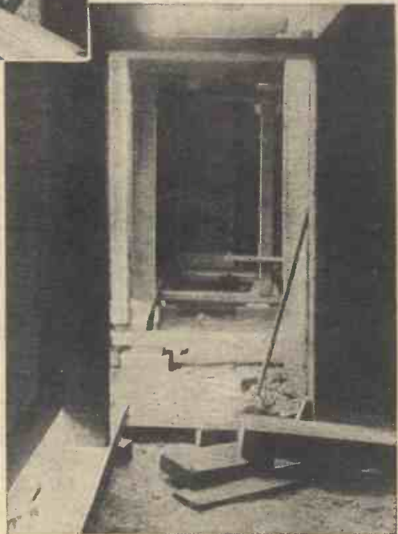
An air-raid shelter capable of accommodating twenty persons. Note the heavy timbring
