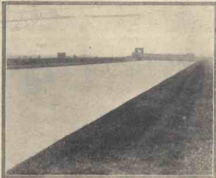
The canal carrying water to the turbines
