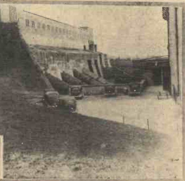
Tubes feeding the turbine and dam for holding back the water
