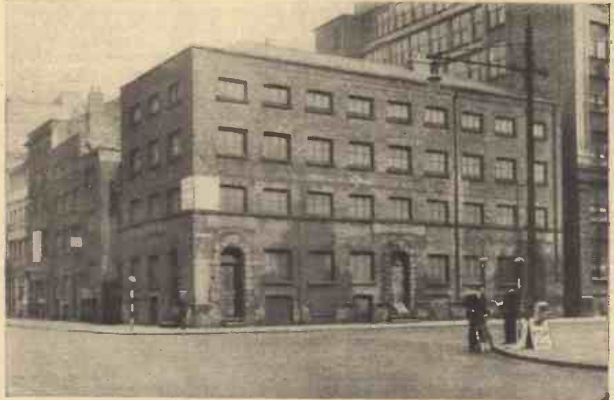
Until recently, this building could be seen in Manchester. It was one of the earliest cotton-weaving mills in the country. In such mills, Cartwright's first looms were employed.
