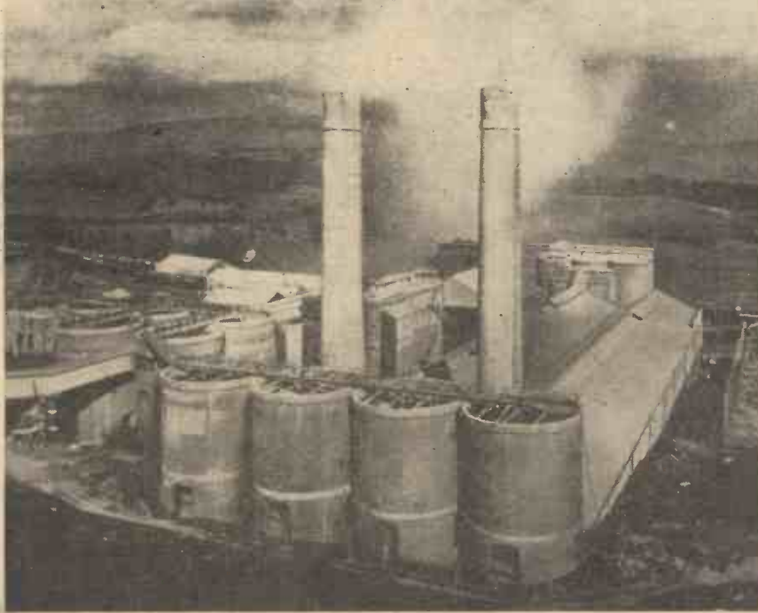
A modern cement works. In the foreground are the slurry thickeners, storage silos are at the back. The two long low buildings on the right house the rotary kilns.
