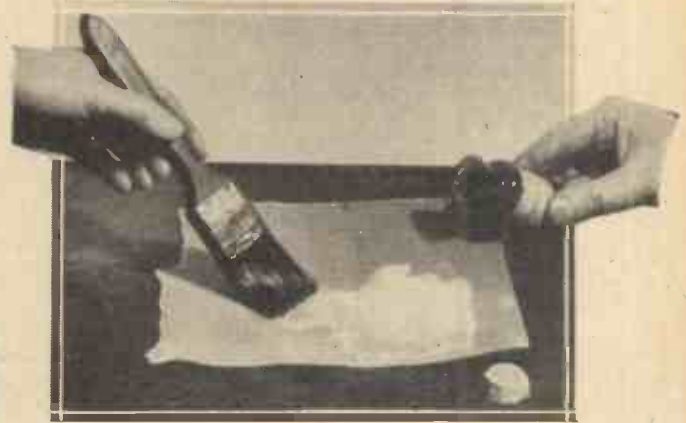
Coating a fine glass paper with luminous calcium sulphide paint.
