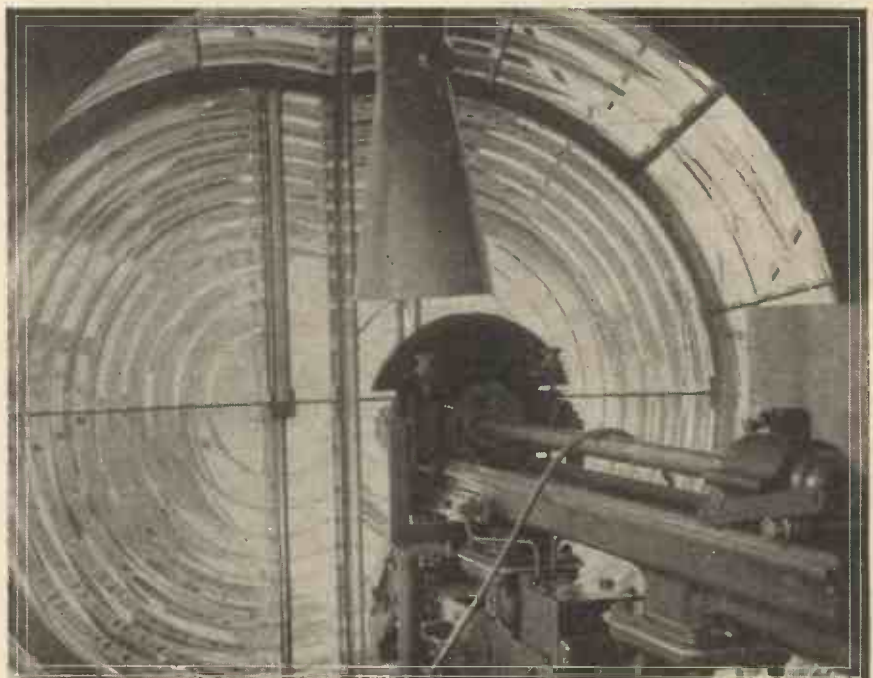
An interior view of the 500 million candle-power lamp constructed for the Creach d'Ouessant Lighthouse.
