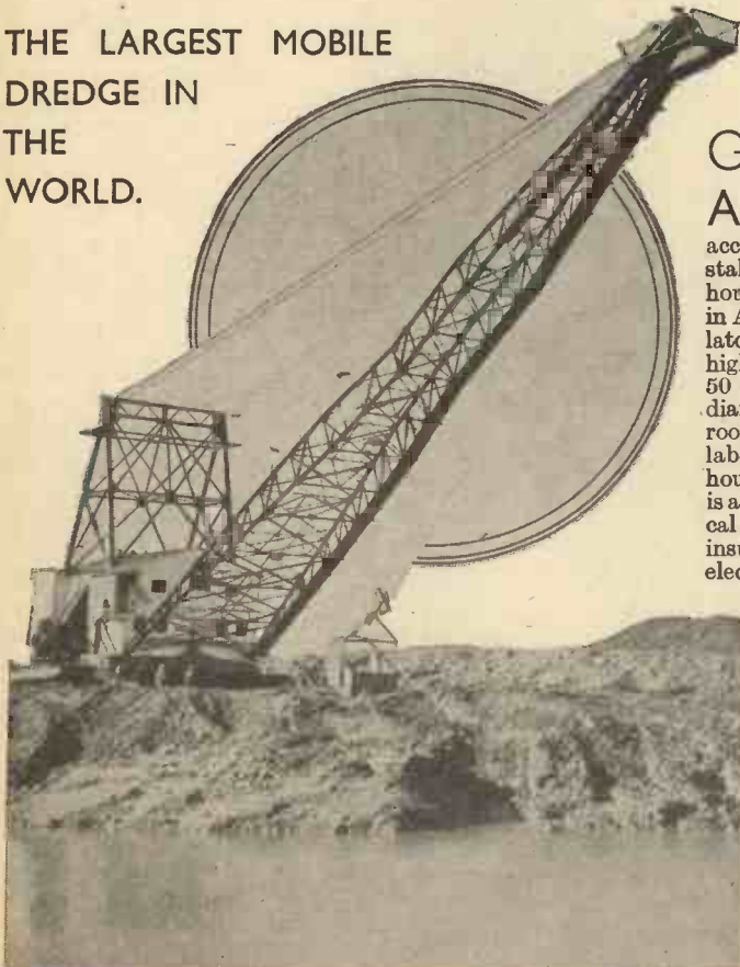
The Mourghan Drag Line dredge, said to be the largest mobile dredge in the world. It is shown at work on the 11,000,000 dollar Ballona Channel Control Government project, to carry off rain water from the motion picture city, Culver City, California.
