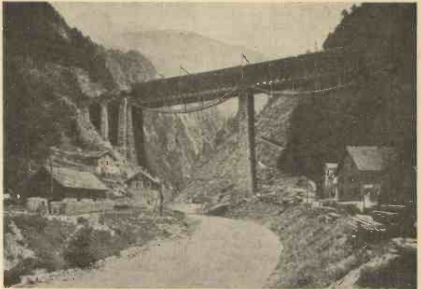
Kerstelenbach Viaduct, St. Gotthard.
