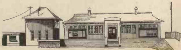
Ramp and stairway approach to platform.
