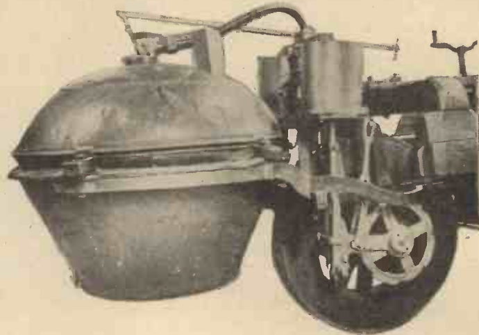
A close-up view of the boiler, cylinders, and piston mechanism of Cugnot's locomotive.
