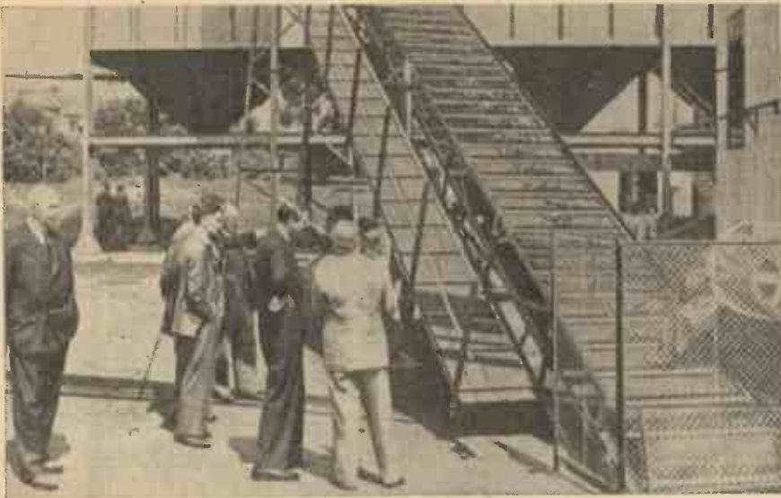
The Duke of Kent watches the briquette elevator at work at Erith.
