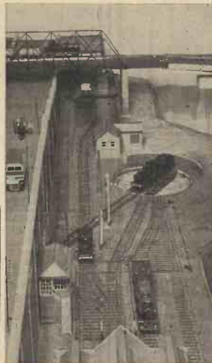
Fig. 4.—A high and stepped-down retaining wall at Laurencetown Old Station W.M.R.
