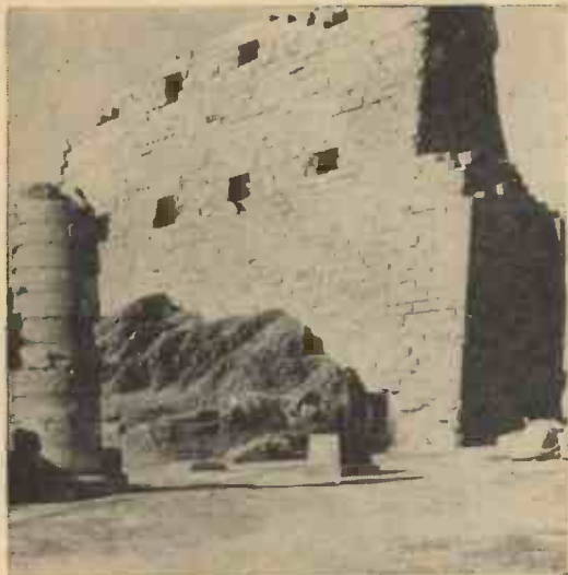
Original scaffolding at Karnak.
