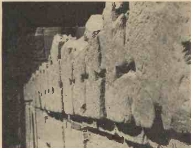
Top of the wall at Karnak showing slots for brass clamps.
