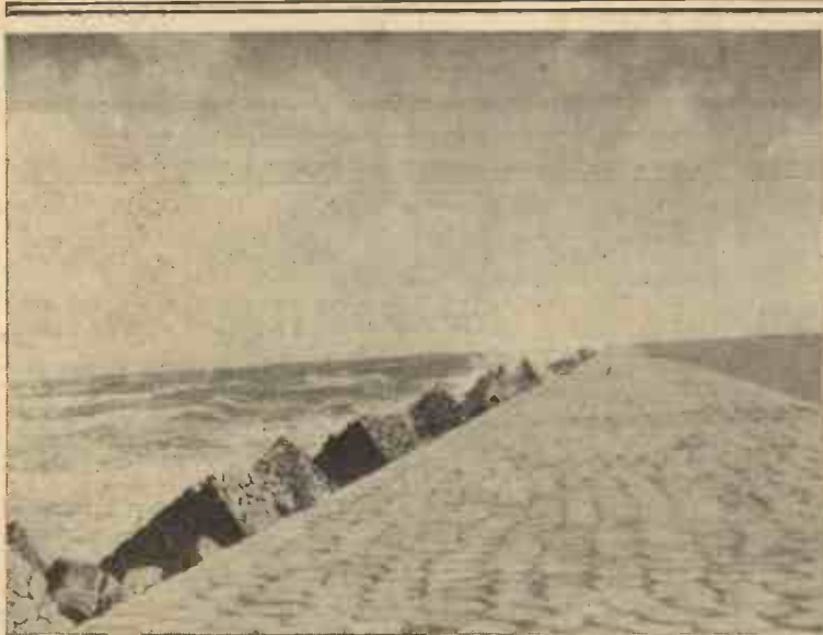
(Left) The West Break-water, three and a half miles long, protects the canal from shifting sands, and is itself a mighty achievement.
