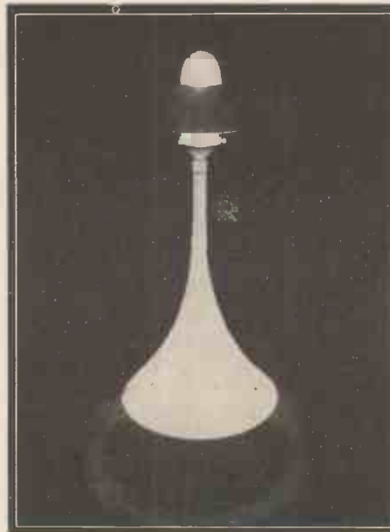
A night view of the new cone-type boundary light at Croydon Aerodrome.
