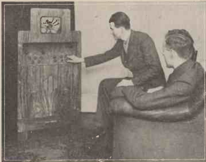
Fig. 4.—A combined vision and sound receiver employing a cathode-ray tube.
