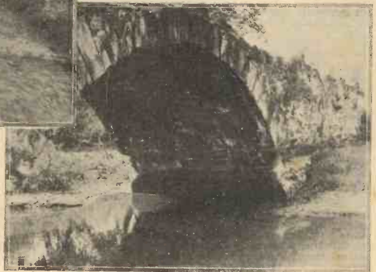
(Right) The Kings Bridge, Panama, over which the incas gold was carried; relic of 1635.
