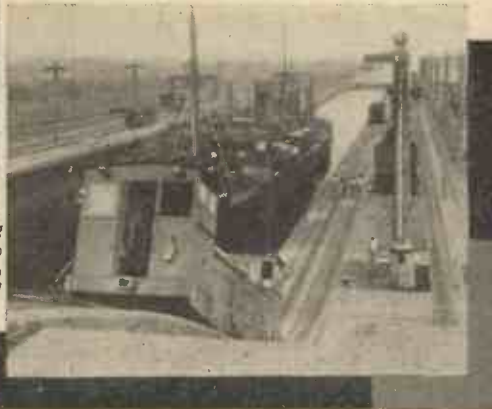
(Above) The Panama railway crossing Rio Chagres. (Right) Towing a ship through Gaton Lock. The electric loco is seen climbing to the level of the second lock (four locos are used to each vessel).
