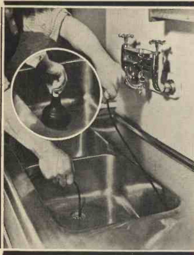
Showing two methods of clearing a blocked sink—first by means of a length of cane, and (inset) by means of a force cup.
