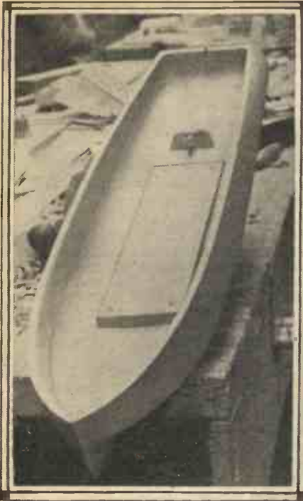
The hull ready for fitting in the steam plant with false floor and stern tube.
