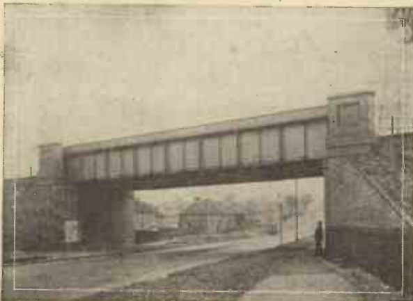
Fig. 10.—A large plate girder carrying a railway over the Sutton By-pass.
