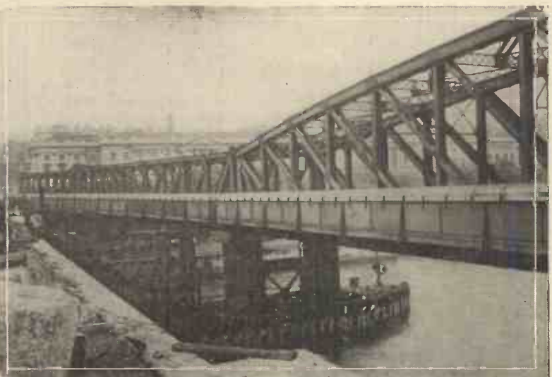
Fig. 13.—The large steel framed girders used for the temporary Waterloo Bridge over the Thames. The bottom booms are hidden by the parapet to the footways.
