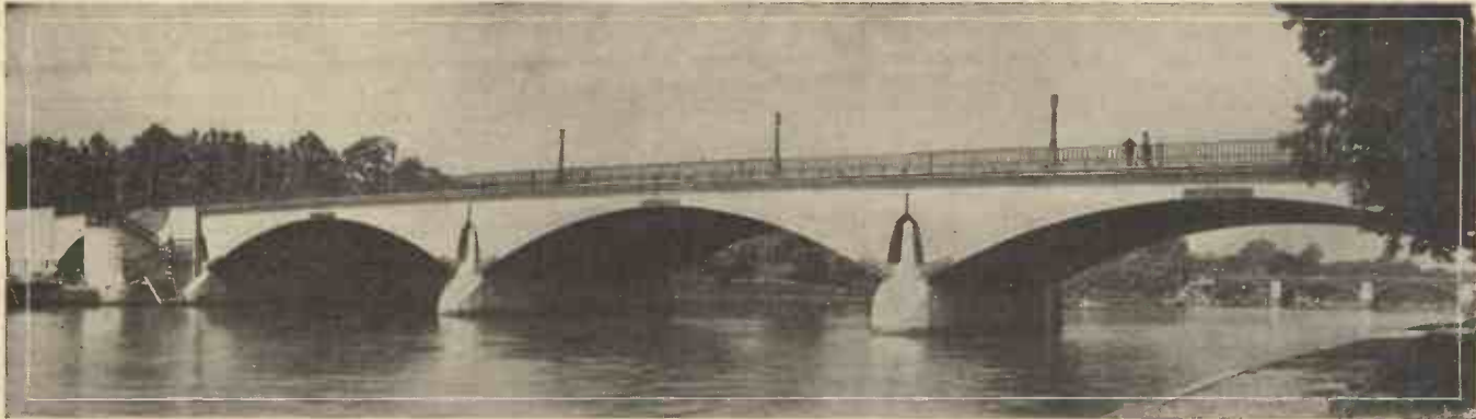
Twickenham Bridge over the Thames, a fine example of a reinforced concrete arch bridge.
